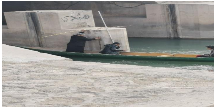
Figure 4 Survey work using Level and the boat to survey the inside of the canal.
