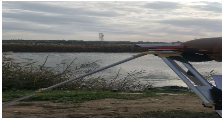
Figure 5 Survey work using a level device.
